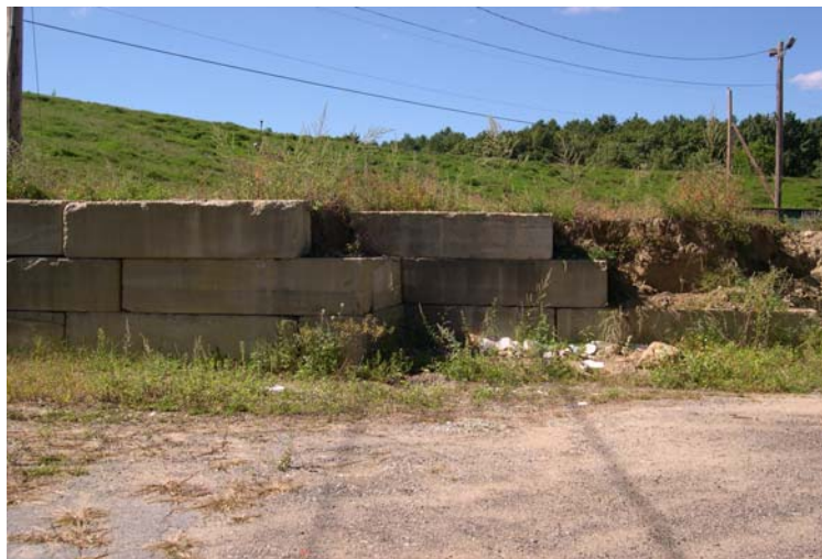
Existing Solid Concrete Block Wall at RCTS Site
