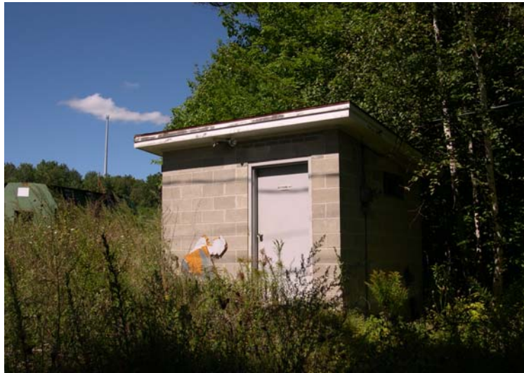
Existing Restroom at the RCTS Site
