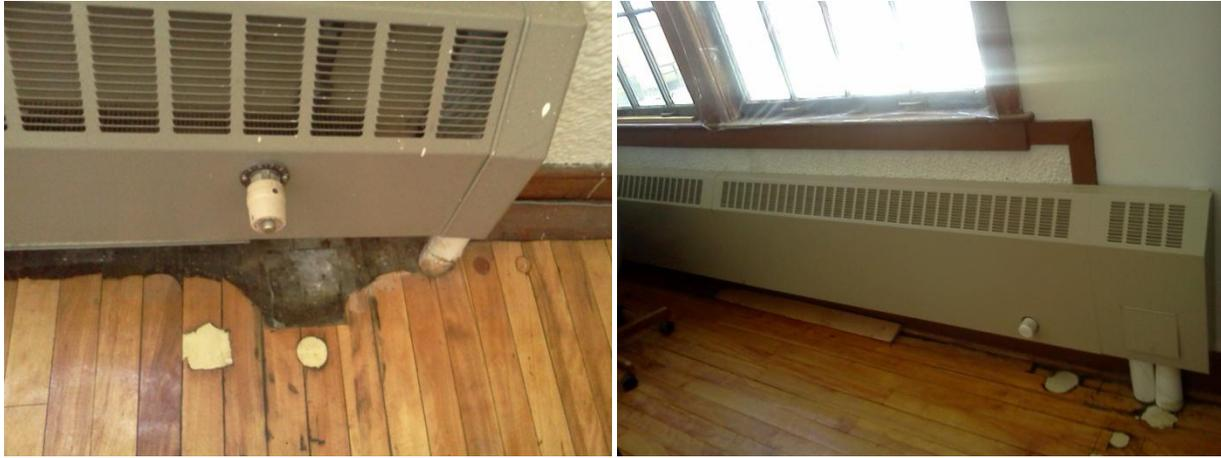
*2: Fin-tube heating elements in the Town Office Building (left- first floor, right - second floor)*
